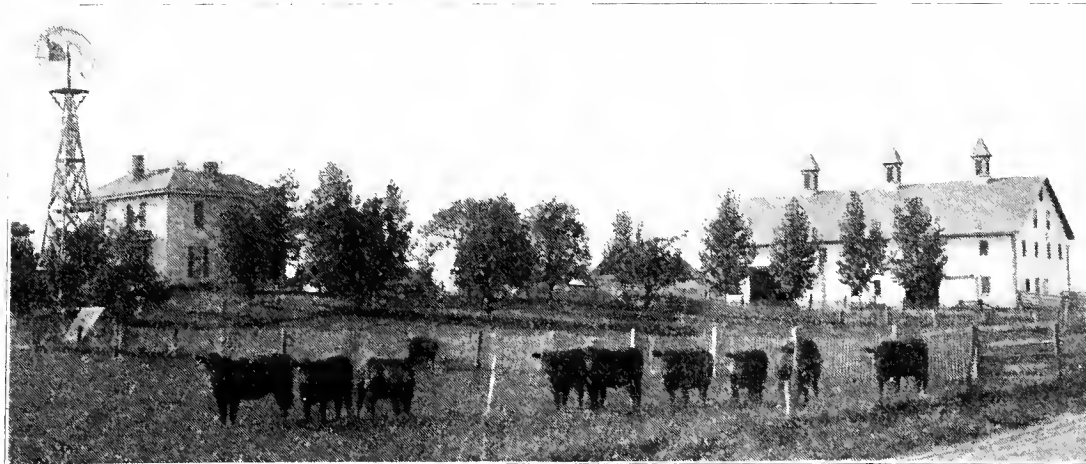
THE YARD AND MAIN BUILDINGS ON THE FARM OF W. R. COFMAN, FAIRFIELD CO., OHIO.
